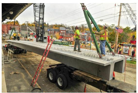
Workers rig straps from a large crane to the first of the new bridge supports put into place over Cobbossee Stream in downtown Gardiner in October. A commission formed to recommend new funding options for transportation projects will ask for more time to draft a long-term solution. *Joe Phelan/Kennebec Journal* Buy this Photo
