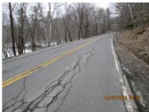
Route 4 Phillips and Madrid, Maine Federal Project STP-1824(700)X Work ID Number 018247.00
