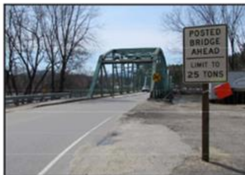
Bridge Number 2019 Federal Project STP-1849(800) Work ID Number 018498.00
