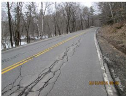
Route 4 Phillips and Madrid, Maine Federal Project STP-1824(700)X Work ID Number 018247.00
