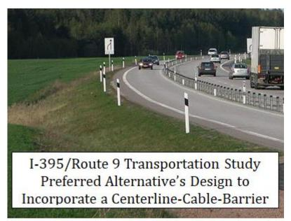
A centerline-cable-barrier separating lanes on a 2+1 road in Sweden. http://en.wikipedia.org/wiki/Cable\_barrier
